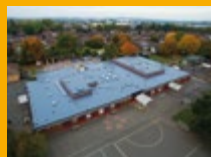
LIQUID APPLIED ROOFING
